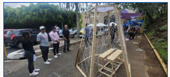
Constructing to full scale
